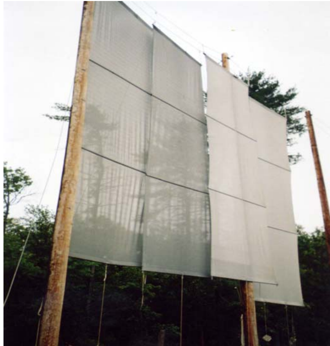
Figure 4: Photograph of Lead Shot Curtain Structure at the Standish Sportsman’s Association Range, East Bridgewater, MA
